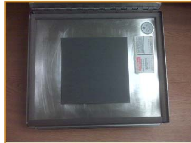
Fig 1d – Inside view showing application of ARC material
